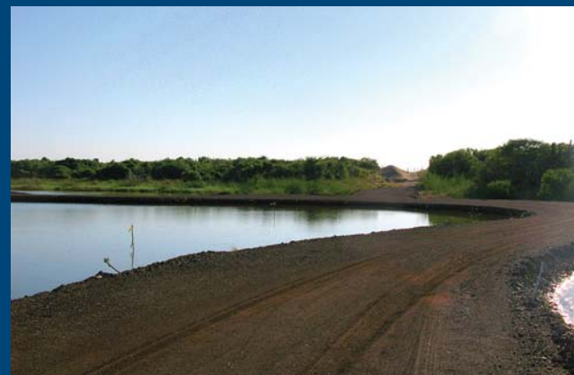
Base road to the property
